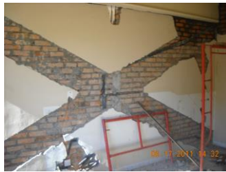
(a) pembobokan plaster dinding bata
