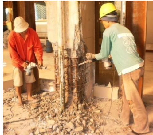
(c) pembobokan beton
