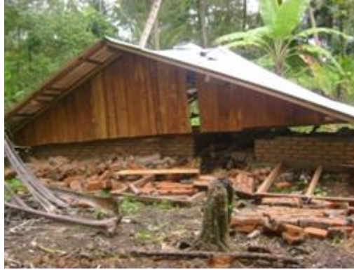
Gambar 6. Dinding bata roboh total
